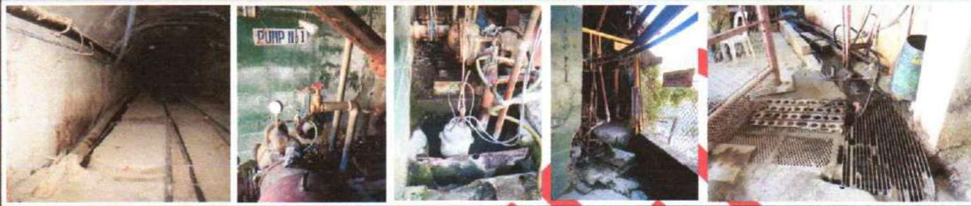
**MOTORPOOL** Oil-water separator built in motor pool workshop/garage that "de-contaminates" used water. Collected used oil from separator is stored in a hazard waste container to be disposed appropriately
